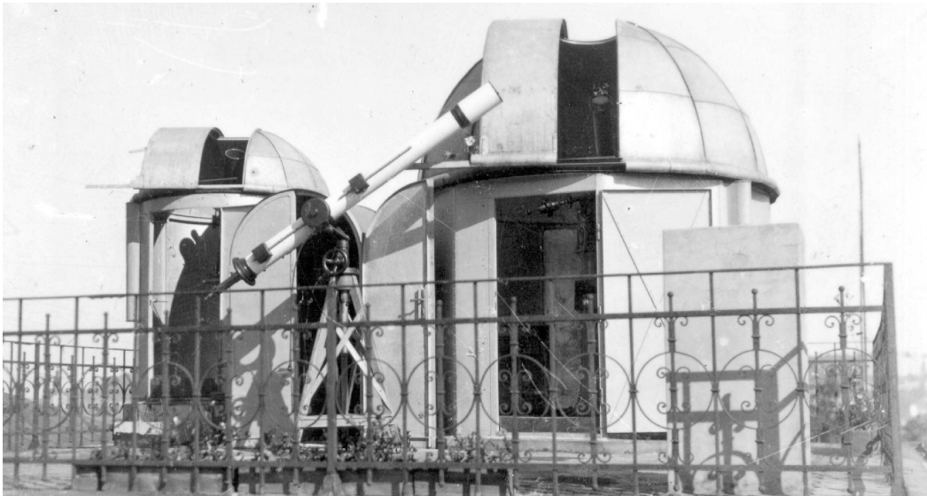
FIGURE 6. The roof observational site with pavilions for telescopes.
